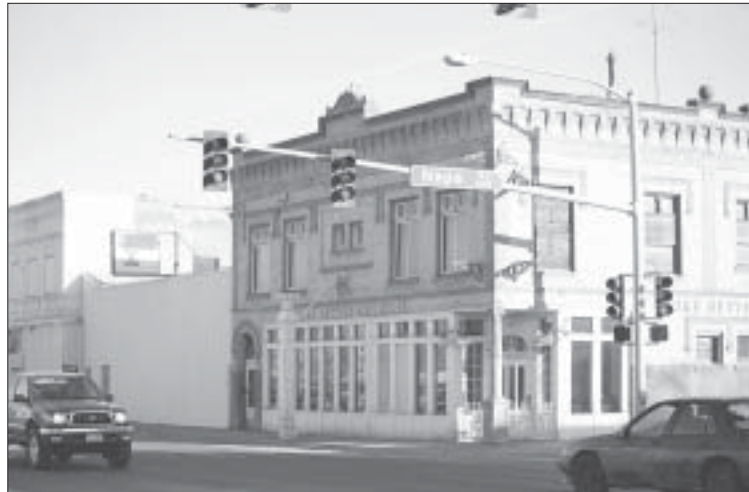
Many East Sprague businesses abut empty buildings.
